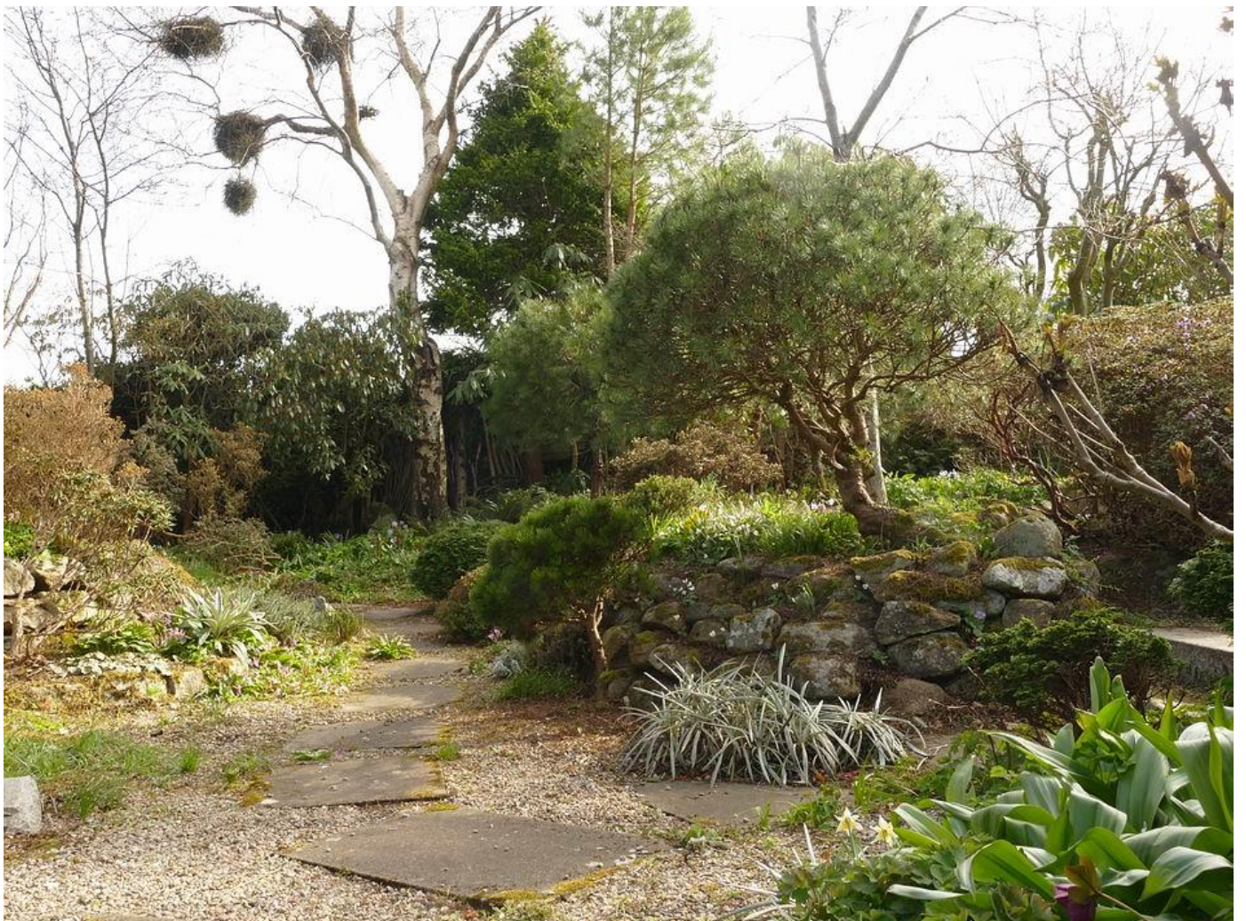
This view of the wall from the high side shows the sides are not vertical but have a slight slope.
